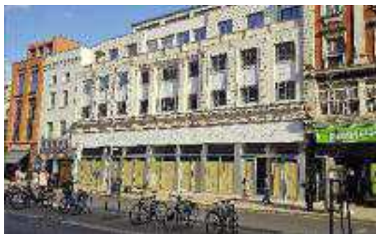
The former Woolworths store after renovation.
