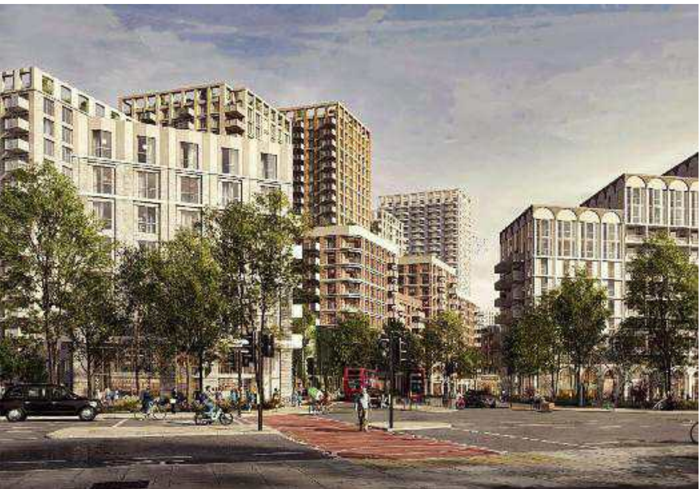
Entrance to the Ballymore-Sainsbury's site by Ladbroke Grove.
