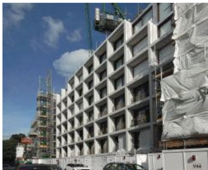
the redevelopment of de Vere Gardens
